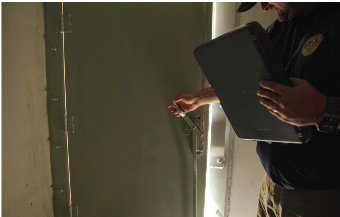
(Safe room Coordinator Kevin Wade inspecting a safe room)
