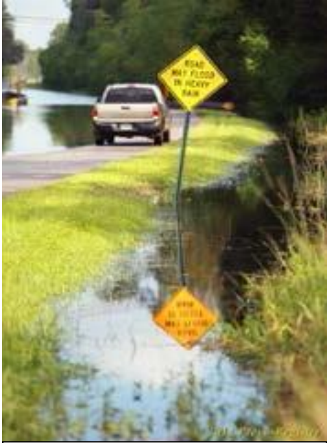
Severe Storms and Flooding, Clarksdale 2016
