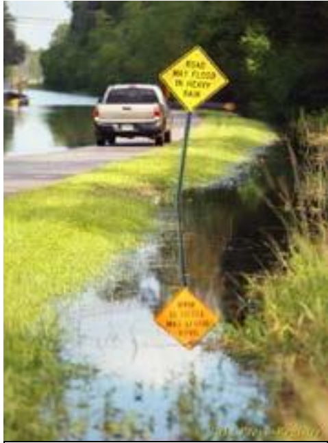
Severe Storms and Flooding, Clarksdale 2016
